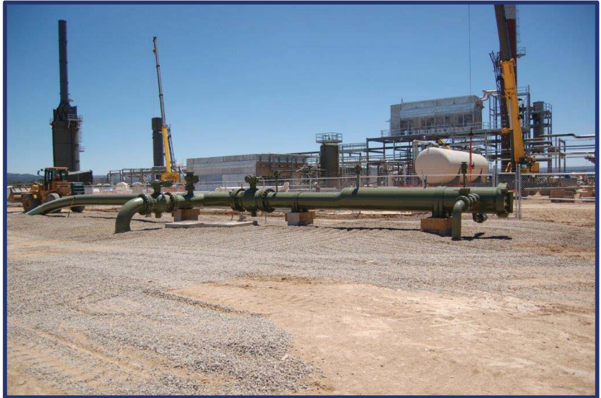
Figure 1.2.4 – Typical Pipeline Pig Receiver / Pig Launcher
