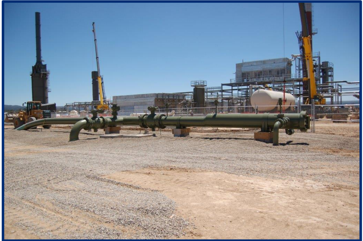
Figure 1.2.4 – Typical Pipeline Pig Receiver / Pig Launcher
